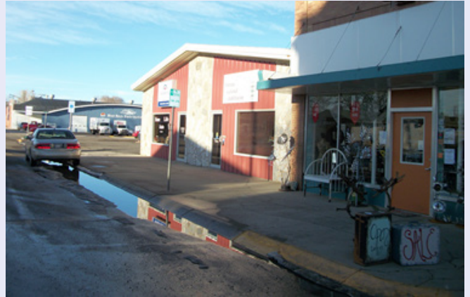
Lack of accessible parking
